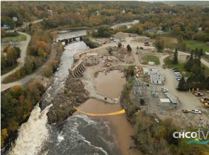
Dam removal in process Photo: CHCO TV
